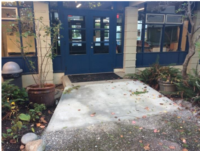
Our new access ramp to the Courtyard
