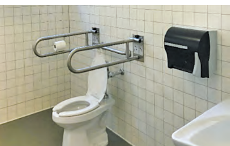
Accessible washroom upgrade at Capilano Elementary
