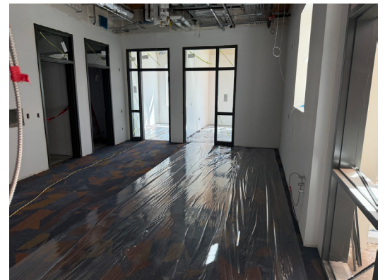
Interior construction progress, April 2026
