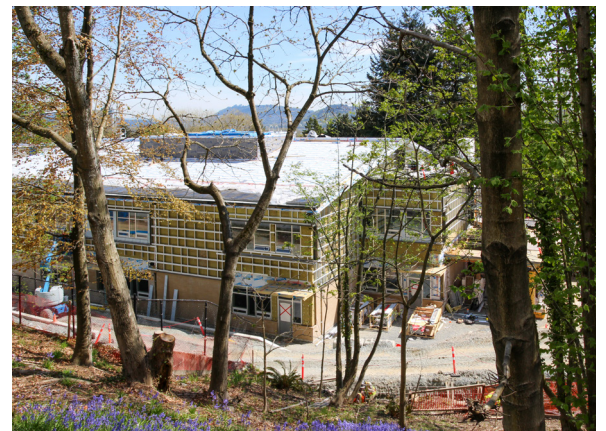
Exterior construction progress, April 2026
