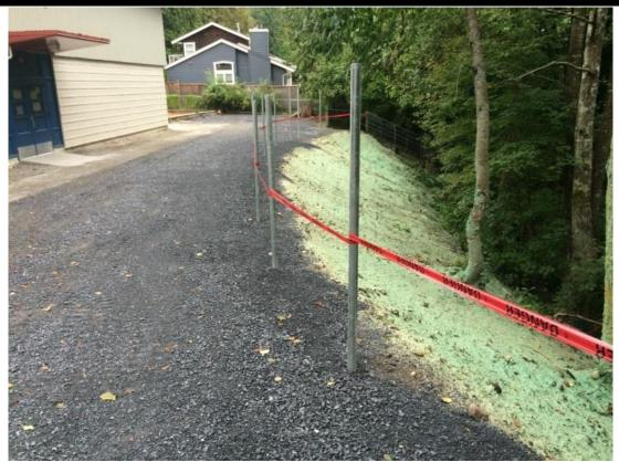
Due to erosion issues, the embankment at the south side of the school went through a remediation process over the summer, where 50 cubic yards of fill were removed, the slope regarded, and new ground cover and fencing was installed. This was a safety issue that needed to be addressed
