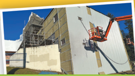
Windsor Secondary receives an envelope upgrade which includes new glazing and siding.
