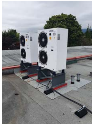
New supplementary electric heat pumps
