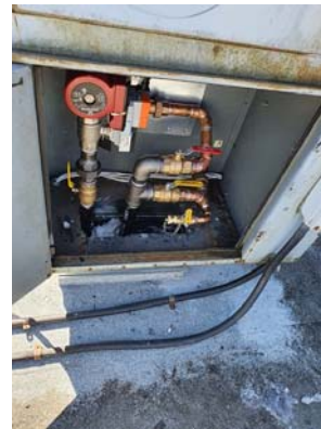
New hydronic coils in rooftop units
