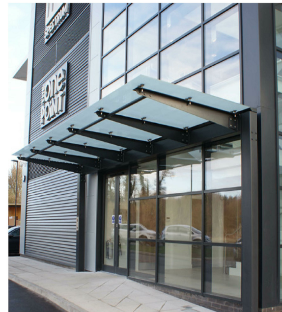
GLASS CANOPY AND PAINTED STEEL STRUCTURE
