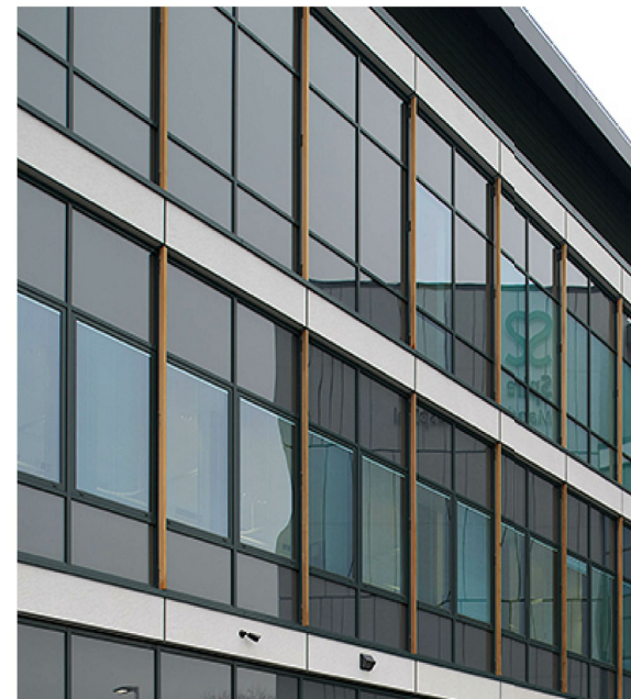
OPAQUE GLASS SPANDREL PANELS
