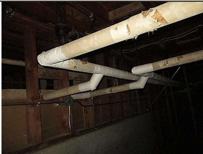
Photo 15 | Location: Crawlspace Description: Non Asbestos Containing Pipe Insulation (Fibreglass)
