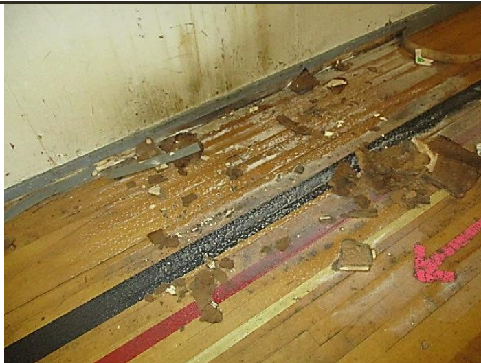
Photo 23 | Location: Gymnasium Description: Mould Growth on Walls & Water Damage
