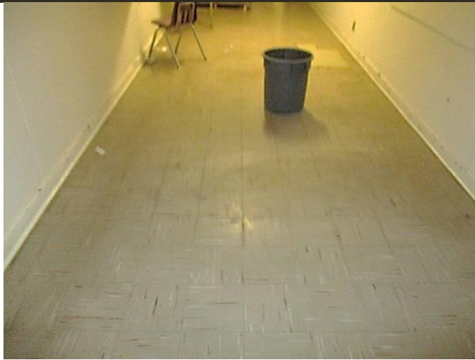
Photo 13 | Location: Basement – Corridor 001 Description: Asbestos Containing 9"x9" Vinyl Floor Tile
