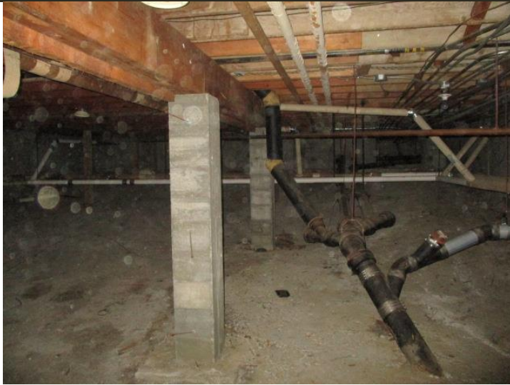
Photo 21 | Location Crawlspace Description: Bell & Spigot Housings (Typical)
