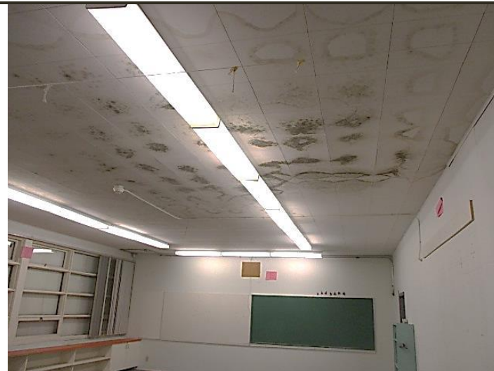
Photo 24 | Location: 1 st Floor – Classroom #3 (117) Description: Mould Growth on Cellulose Ceiling Tiles
