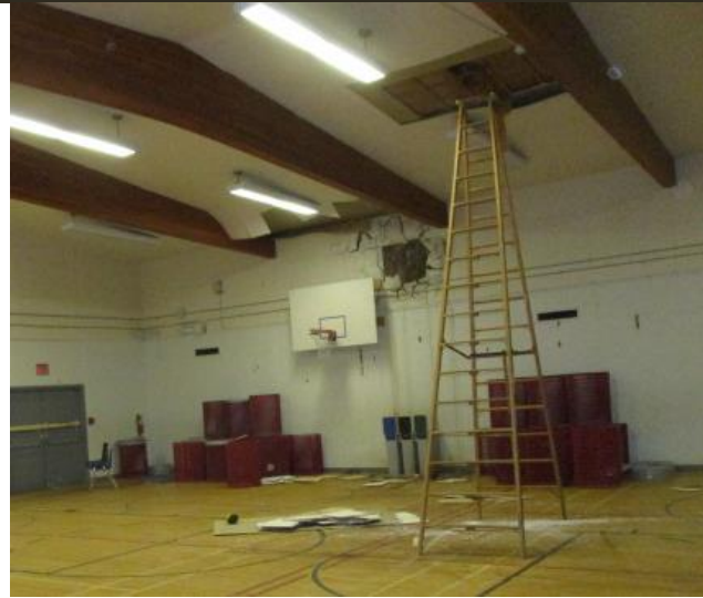
Photo 22 | Location: Gymnasium Description: Water Damage to Wall & Ceiling
