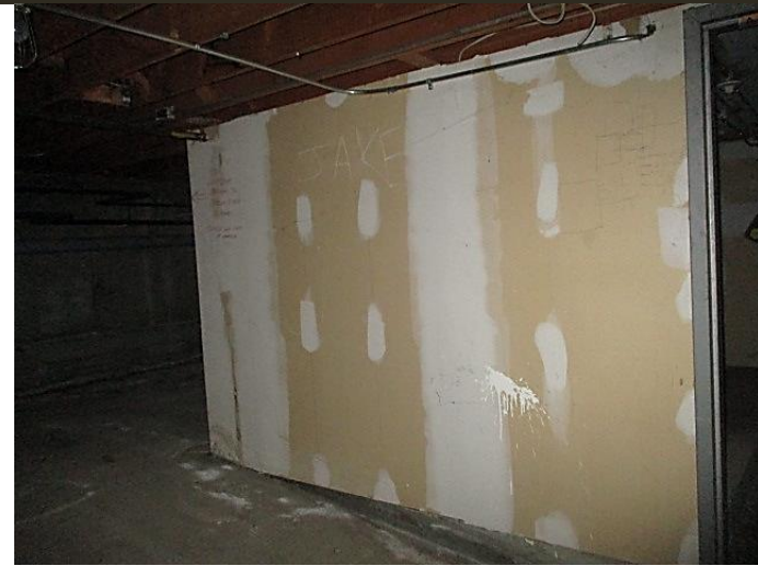
Photo 14 | Location: Low Height Storage in Basement Description: Drywall Joint Compound (Treat as asbestos)
